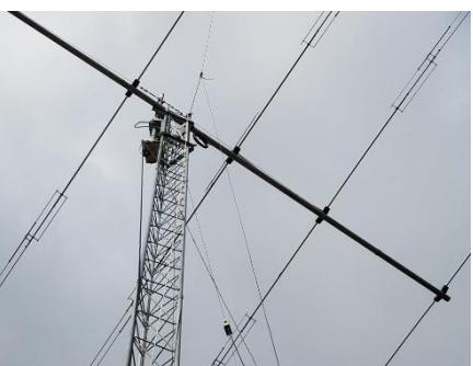
The antenna is fed with 50 ohm coax and the center insulator is not using any balun or choke. With some minor adjustment to the
